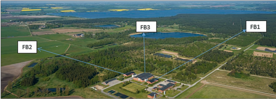
Figure 1. Overview of Vombverket water treatment plant with the different filter blocks (FB).
