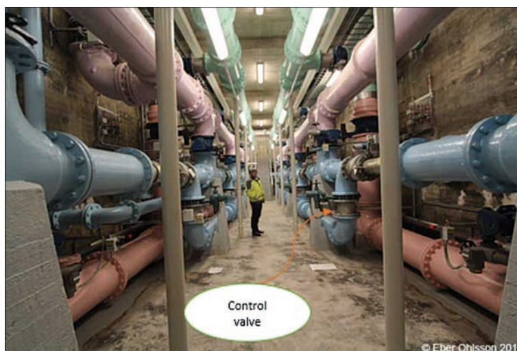
Figure 7. Inside view of one of the filter buildings, where blue pipes carry filtered water, orange pipes are for drainage, the green upper most pipes are feeding the filters with raw water, and the pink pipes are for backwashing the filters.
