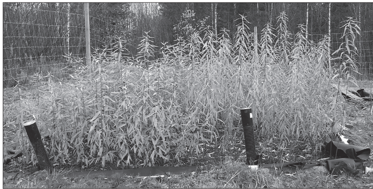
Figure 2. Pre-treatment step – gravel bed planted with willows, Luleå (Rastas, 2006).
