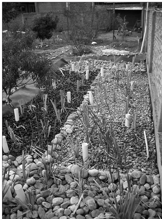
Figure 1. The HSF constructed wetland PTAR1. The black part is the plastic medium and the white tubes are observation pipes.
