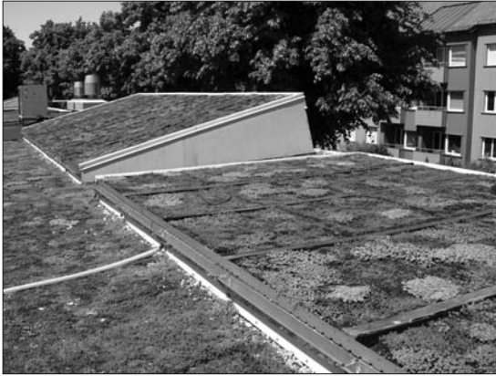
Fig. 1. Green roof – sampling point 1.
