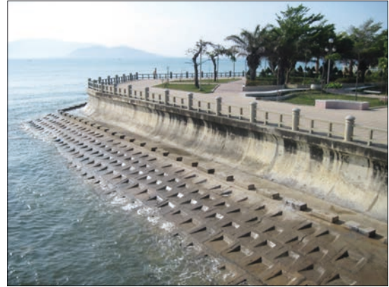
Figure 3. Concrete construction around Yersin Park at the river mouth of Cai river.
