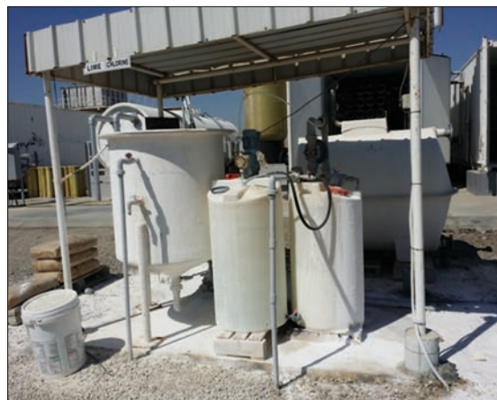
Figure 3. Left panel: an example of deep wells intake for desalination plant. Right panel: treatment point for the pH and chlorination balance.
