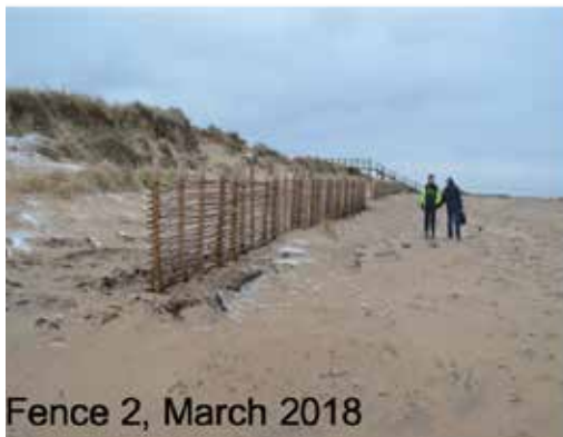
Figure 5: Pictures showing the seasonal differences in sand accumulation along the sand fences on Vejbystrand during 2018. Fence 1 in March 2018 is seen in the top left corner. The same fence is seen in September 2018 on the top right. Fence 2 in March 2019 is seen on the bottom left and the same fence is seen in September 2018 on the bottom right. The pictures taken in March are by the author and the pictures from September are taken by Geraldine Thiere, Ängelholm municipality.
