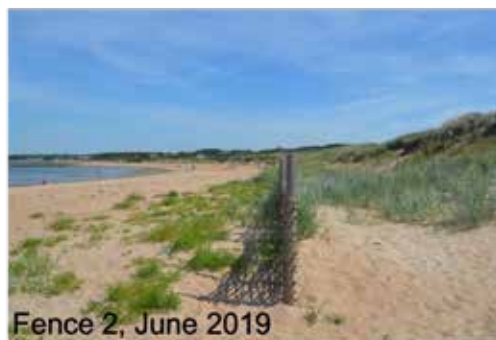
Figure 10: Pictures showing the differences in sand accumulation along the sand fences in Vejbystrand from Summer 2018-2019. Fence 2 in September 2018 is seen in the top left corner. The same fence is seen in June 2019 in the top right. Fence 3 in September 2018 is seen in the bottom left and the same fence is seen in June 2019 in the bottom right. The pictures are taken by the author.
