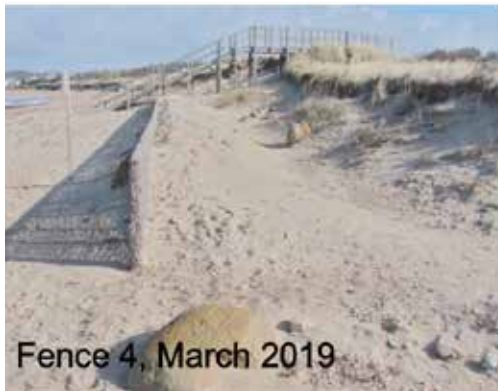
Figure 6: Pictures showing the seasonal differences in sand accumulation along the sand fences in Vejbystrand during 2019. Fence 3 in April 2019 is seen in the top left corner. The same fence is seen in June 2019 in the top right. Fence 4 in March 2019 is seen in the bottom left and the same fence is seen in June 2019 in the bottom right. The pictures taken in June are by the author and the pictures from April/March are taken by Eva Thulin, resident in Vejbystrand.
