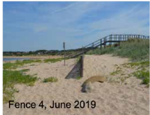
Figure 6: Pictures showing the seasonal differences in sand accumulation along the sand fences in Vejbystrand during 2019. Fence 3 in April 2019 is seen in the top left corner. The same fence is seen in June 2019 in the top right. Fence 4 in March 2019 is seen in the bottom left and the same fence is seen in June 2019 in the bottom right. The pictures taken in June are by the author and the pictures from April/March are taken by Eva Thulin, resident in Vejbystrand.
