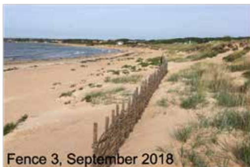
Figure 10: Pictures showing the differences in sand accumulation along the sand fences in Vejbystrand from Summer 2018-2019. Fence 2 in September 2018 is seen in the top left corner. The same fence is seen in June 2019 in the top right. Fence 3 in September 2018 is seen in the bottom left and the same fence is seen in June 2019 in the bottom right. The pictures are taken by the author.
