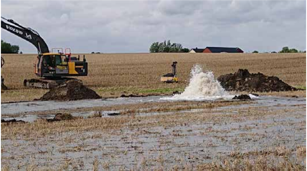
Figure 1. The pipe break that occurred between Teckomatorp and Västra Strö. Photo by Sydsvatten AB.
