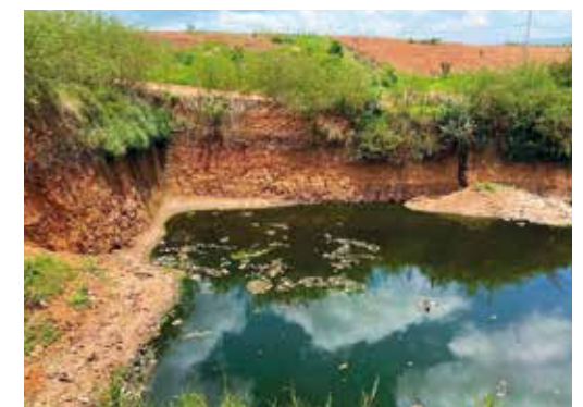
Figure 3. One of the three ponds designated for the storage of leachate water.
