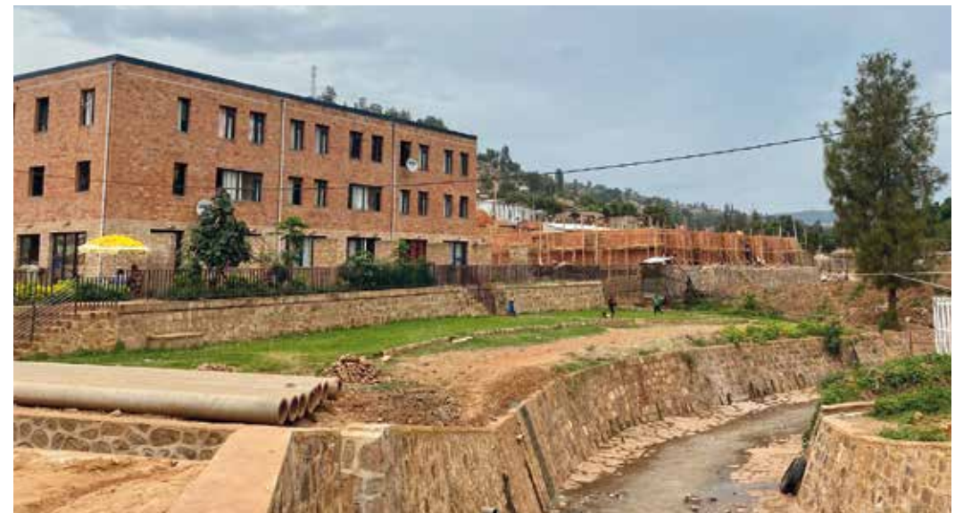
Figure 5. Upgraded main channel in Mpazi neighborhood.
