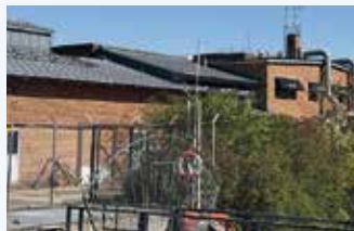
Turbinens pumpstation i Malmö
