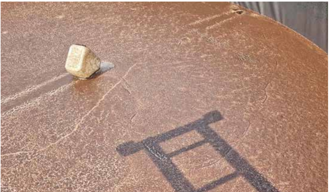
Figure 9. Sludge blanket on top of the sequencing batch reactor (SBR) on the morning of the 3rd of June.
